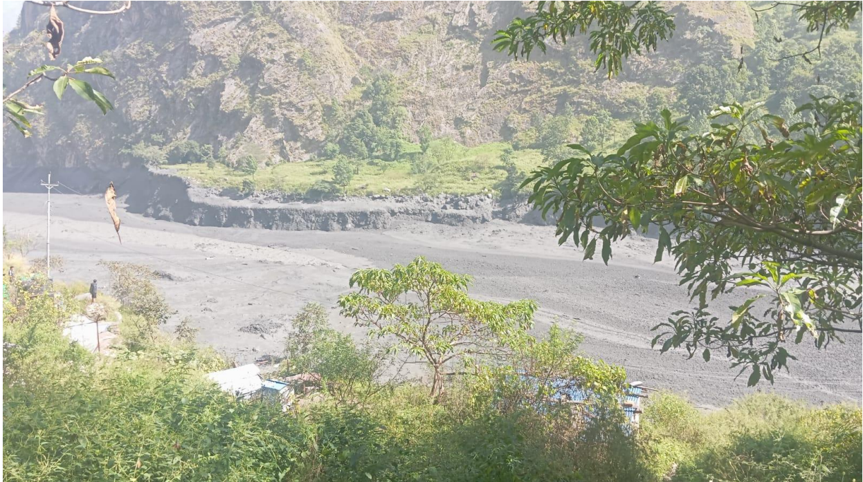
Photo 1. Riverbed buried in grey debris below a settlement, with houses at the edge of the deposit.
