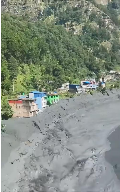
Photo 4. Houses along the riverbank, with the debris deposit reaching their foundations.
