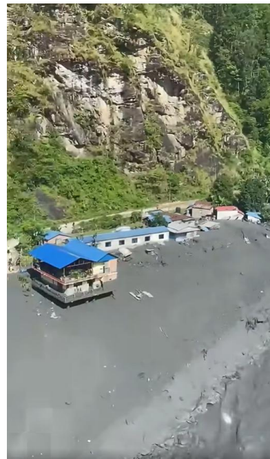
Photo 3. Buildings standing in debris and mud left by the flood.
