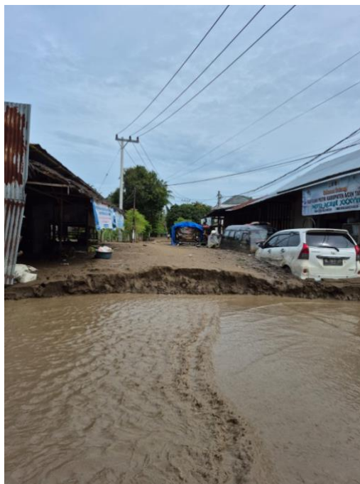
Fig.3.3: Floodwaters and thick mud-covered roads and buildings in Aceh, following the Flash floods
