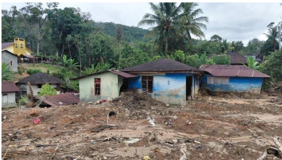
Fig. 1.5: Homes in Tarutung, North Sumatra damaged by flash floods and landslides Photo Credits: YEU Indonesia
